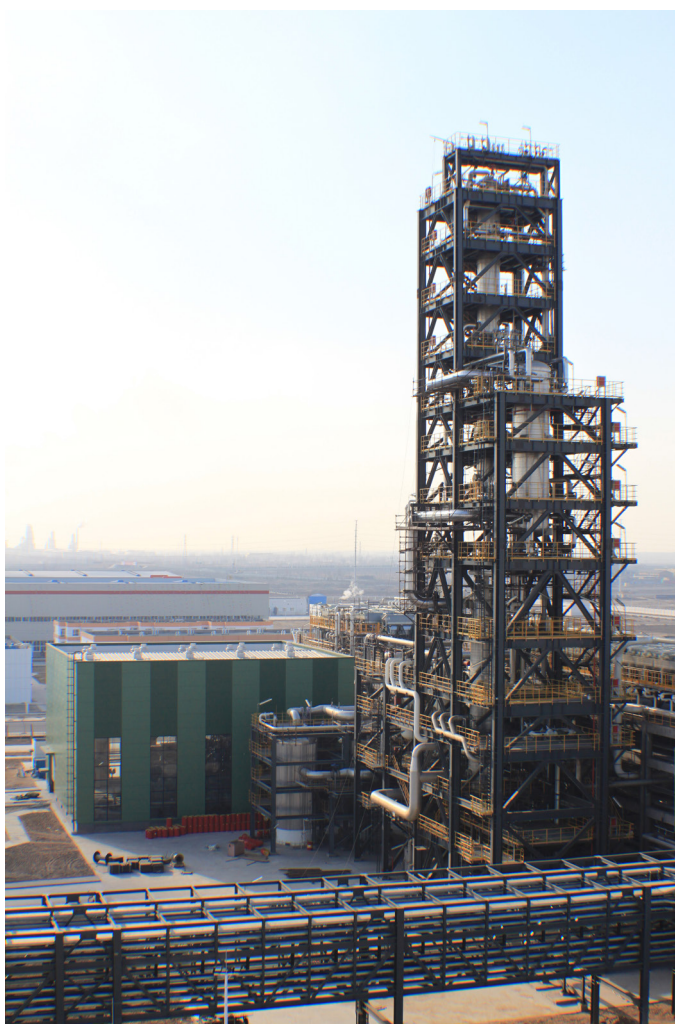
Figure 4. The Ningxia Hanas mid scale LNG plant in China utilises Air Products' AP-SMR™ process.
